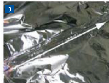
3 Lift the overlap, crease and fold flat for the length of the seam (26 in).
