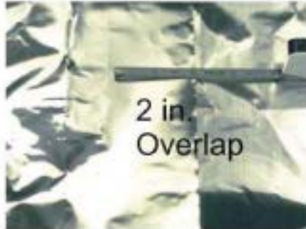
Overlap the two pieces by 2" – lengthwise.
