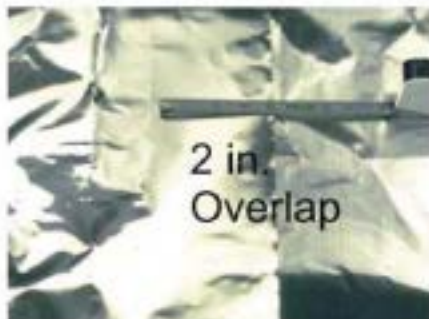
Overlap the two pieces by 2" – lengthwise.
