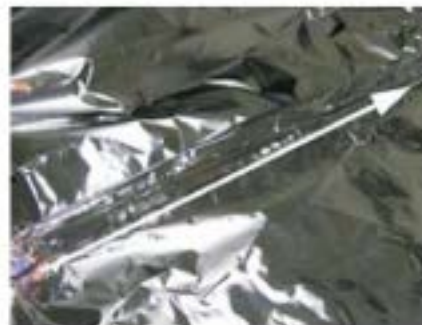
Lift the overlap, crease and fold flat for the length of the seam (26").
