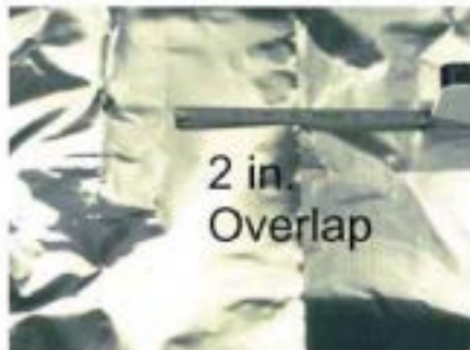
Overlap the two pieces by 2" – lengthwise.
