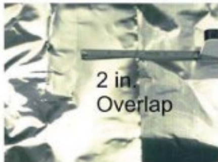
Overlap the two pieces by 2" – lengthwise.
